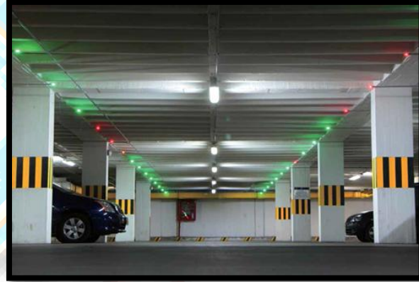
Fig9. Inside of Parking Lot
